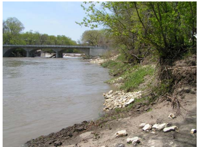
Cottonwood Falls Streambank Stabilization Project Rock vanes are partially submerged due to high water.
