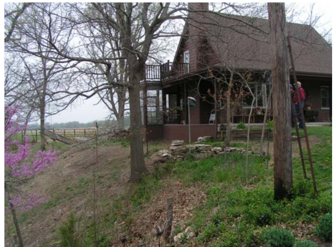
Holt Streambank Stabilization Project, Cedar Creek a tributary to Grouse/Silver Creek Watershed. LAC/FHC Chapter Meeting Tour on 4/23/08
